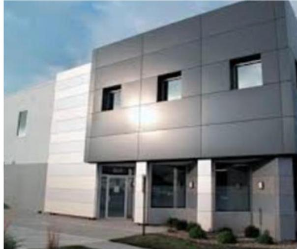
Most composite panels tend to be flat/smooth faced panels like the ones shown above, although some come in profiled form like the one shown below. Once in situ, it can be impossible to tell the insulant without supporting documentation.
